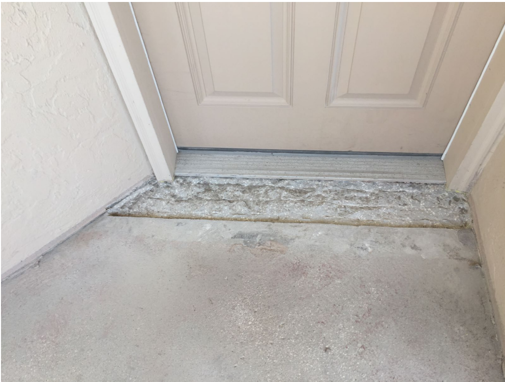
Picture 2: Topping repair at curbs at unit entry doors
