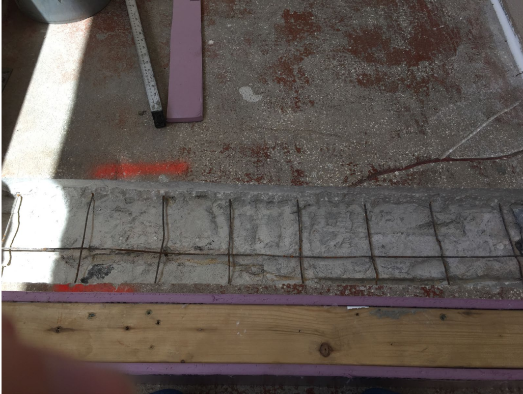
Picture 1: In-progress topping repair
