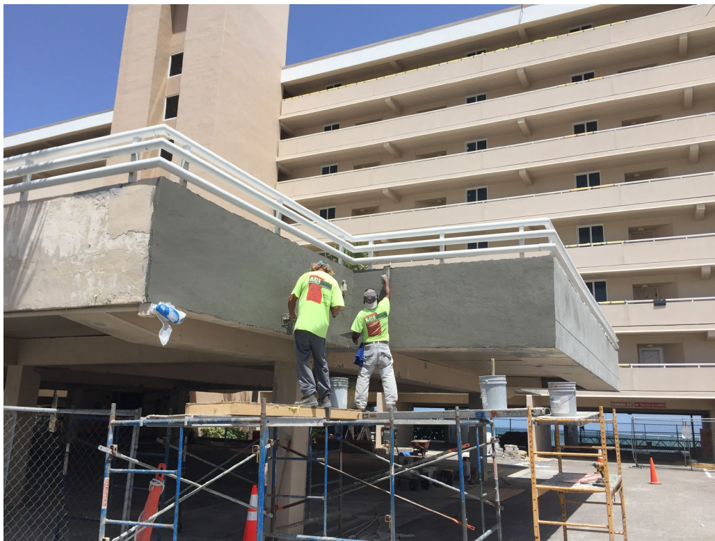
Picture 3: In-progress stucco repair
